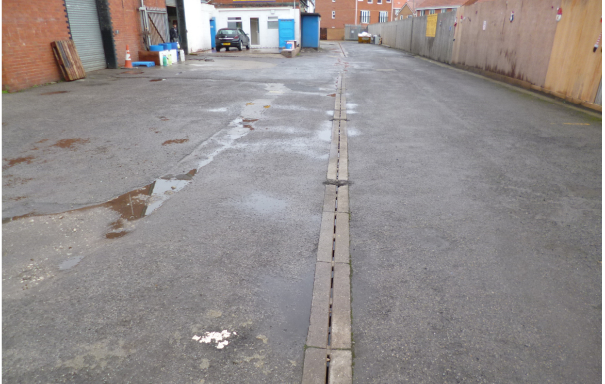
3i) above; view to drainage channels with unit entrance on left 4) below; entrance to valet/storage area where generator is sited
