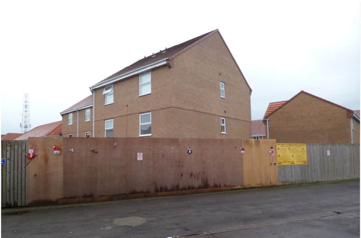
5) above; view to erected 2.6m high panels attached to fence adjacent to 32 Darbyshire Close
